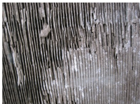
Corroded condensers!
