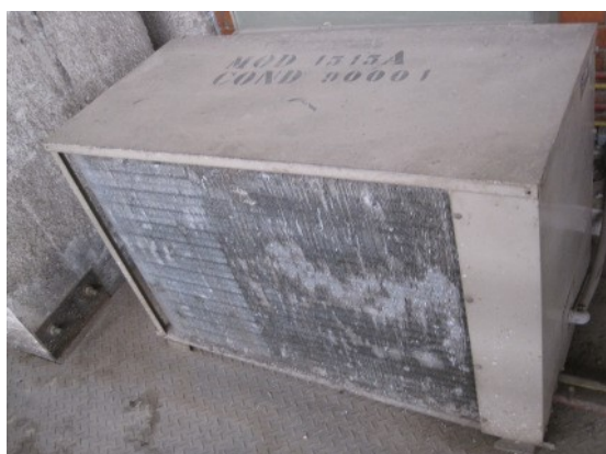
Corroded condensers!
